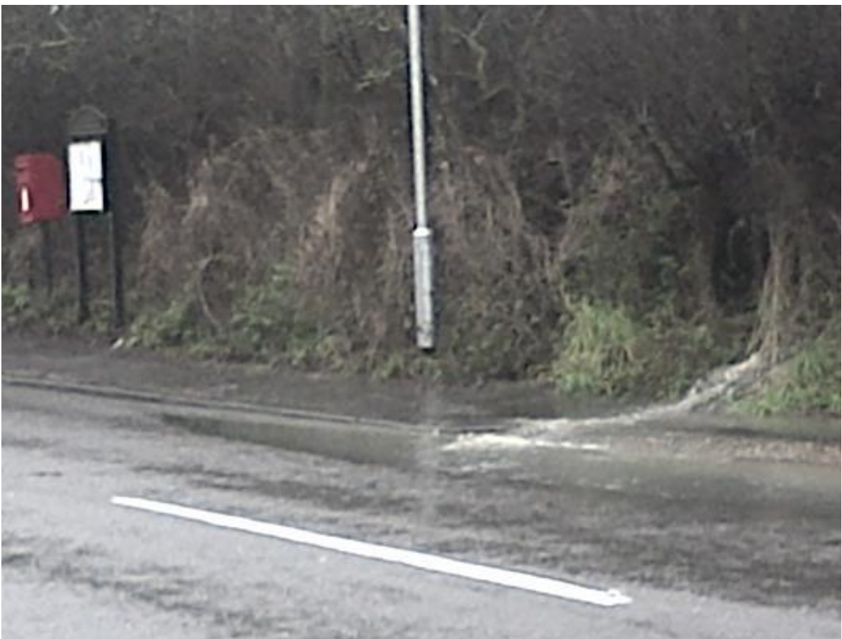
Pound Lane, opposite post box near Kelly Road.
